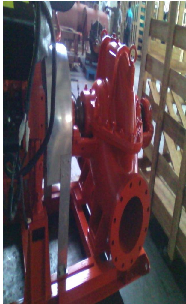
Fig.3. COUPLING OF DIESEL ENGINE AND PUMP
