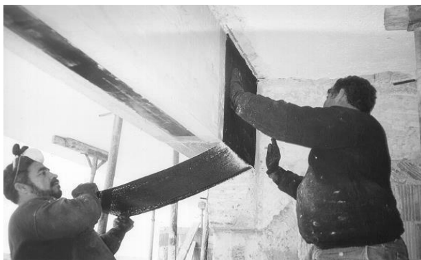
Fig. 1 : Wet lay-up of CFRP sheets
