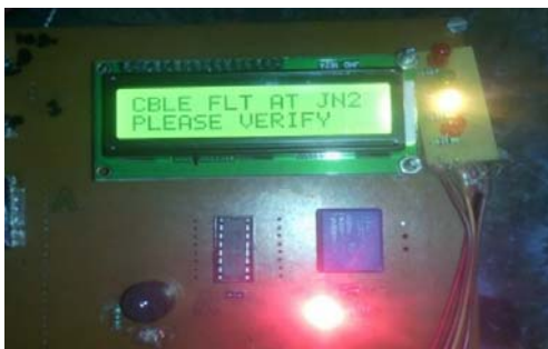
Fig 3. Photograph of underground cable fault detection at junction JN2
