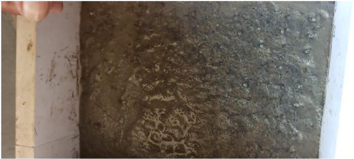
Fig.3.14: placing of concrete
