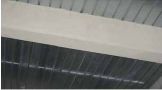
FIGURE 1.4: Steel member with Hand troweling cementitious spray fire proofing
