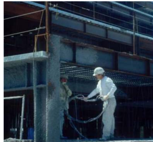
Figure 1.3: Construction worker applying spray resistive material
