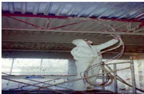
FIGURE 1.5: Spray gypsum based plaster fireproofing being installed.
