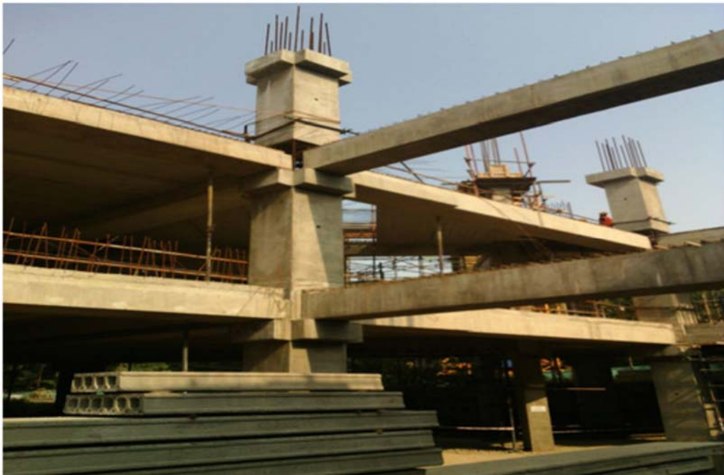
Photograph 1 Internal Column-Beam joint.
