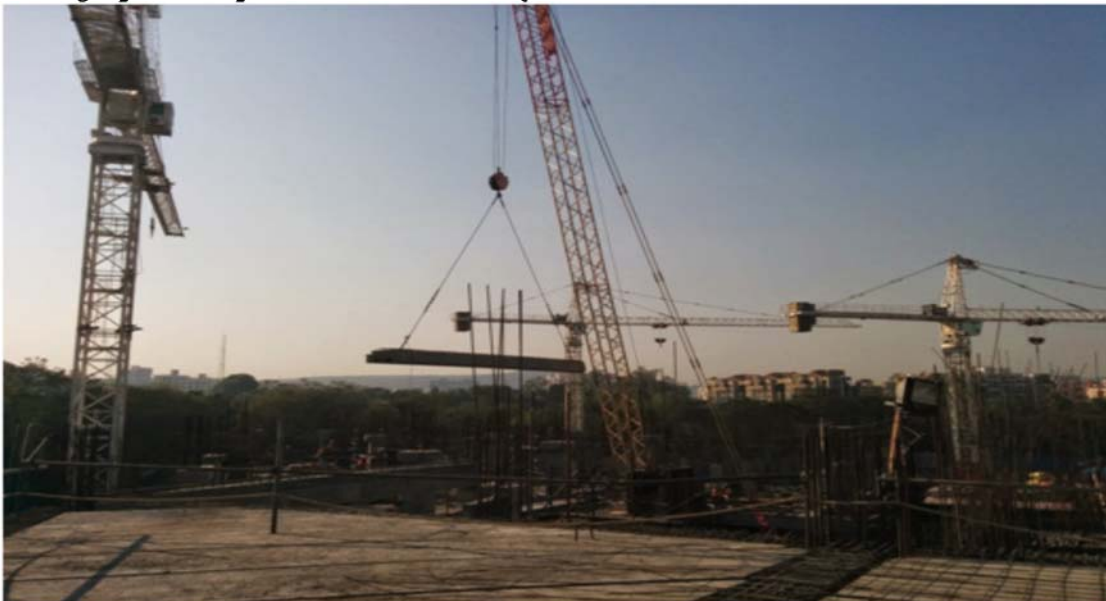
Photograph 3 Installation of Beam
