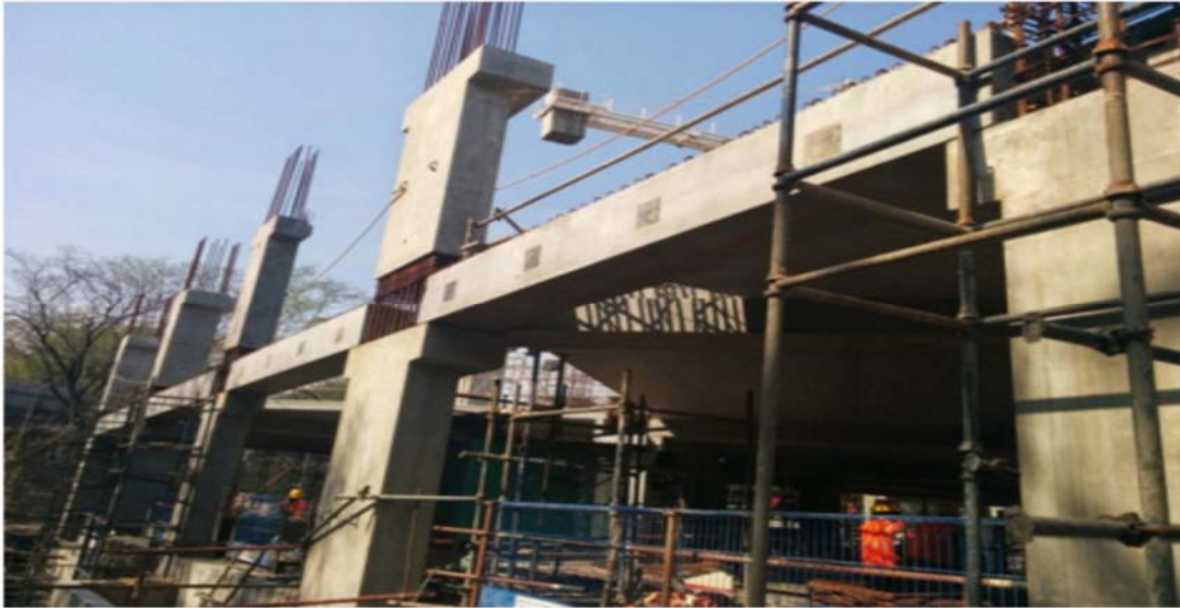
Photograph 2 Peripheral Column-Beam joint.
