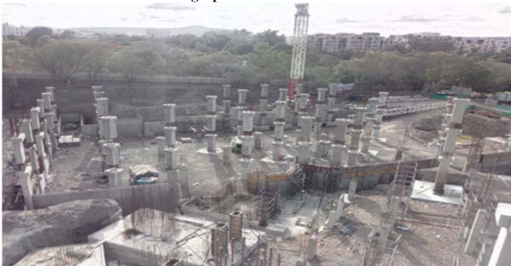
Photograph 4 Site view, Pockets in Column for continuing Beam reinforcement
