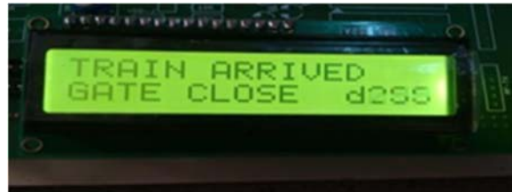
Figure 10. LCD displays the status of gates closed automatically at level crossing
