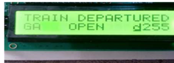
Figure 11. LCD displays the status of the process after the gates opened
