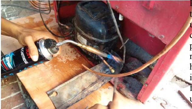
Fig. 2 Brazing Process
