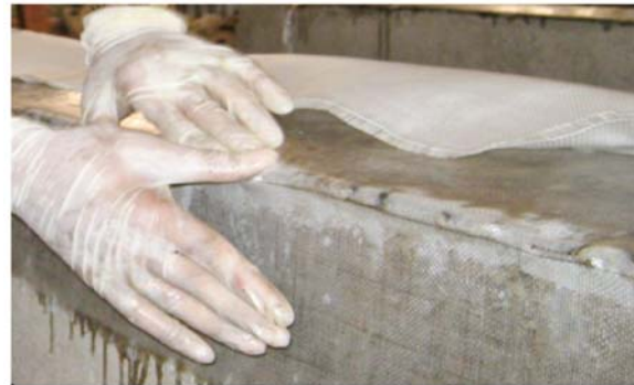
Fig 2.Fixing Of Gfrp Sheets On The Beam
