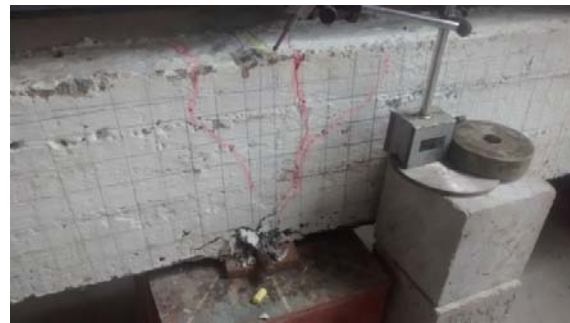
Fig 6. Failure Modes Of Rectangular Beam
