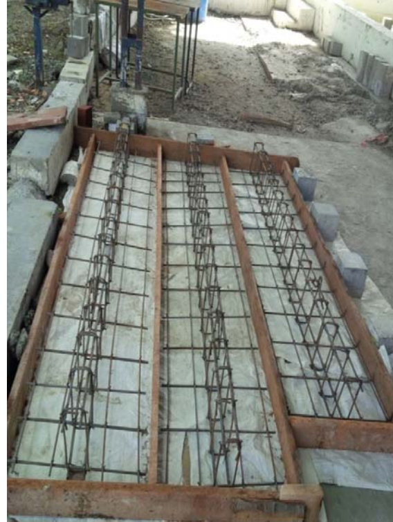
Fig 1.Beams With Their Moulds
