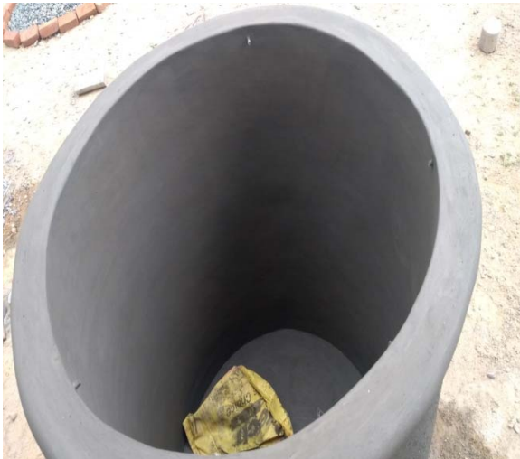
Fig 12. Tank inside finishing
