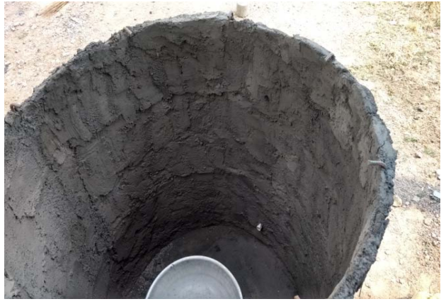
Fig 10. After completion of wall plastering
