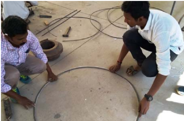
Fig 4. Fabrication of steel
