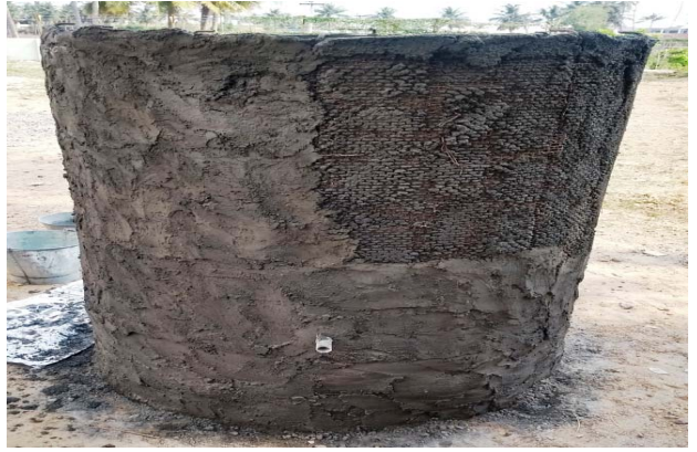
Fig 9. Side wall plastering
