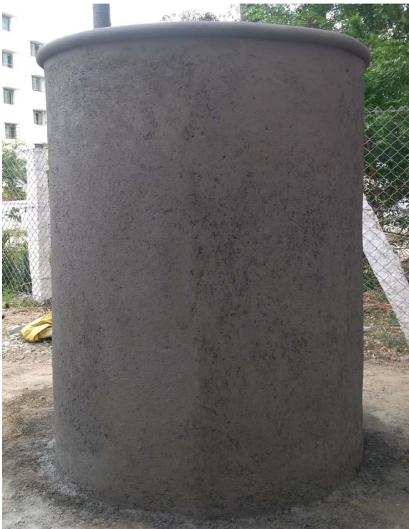
Fig 13. After completion of work
