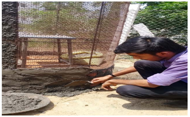
Fig 8. Applying mortar for bottom
