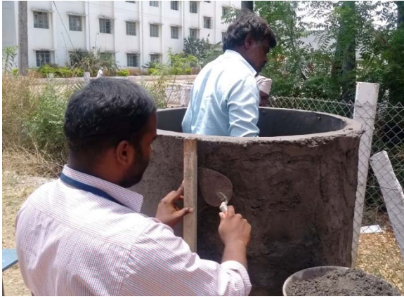
Fig 11. Outside wall finishing
