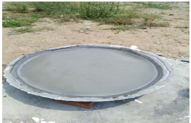
Fig 4. Curing the dome
