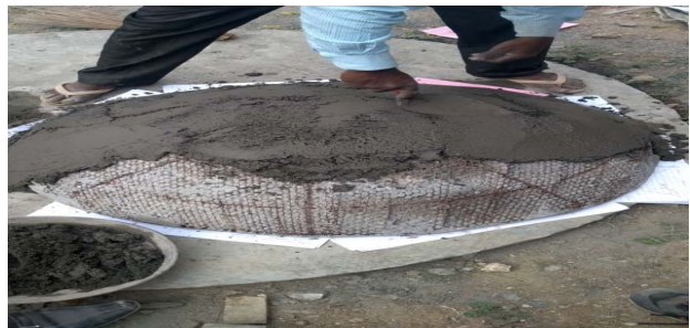
Fig 2. PCC work for dome
