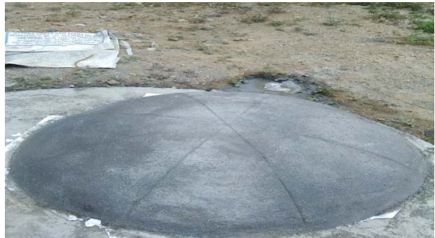
Fig 3. Finishing the dome
