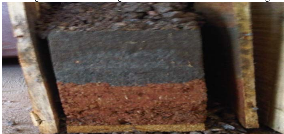
Fig 4: Merging - Improper Separation of sub-grade from the sub-base
