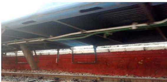
Fig 3.2: Bottom view of disposal pipe
