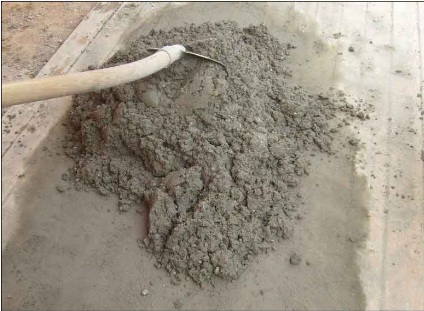
Fig No 4.1: Mixing of concrete
