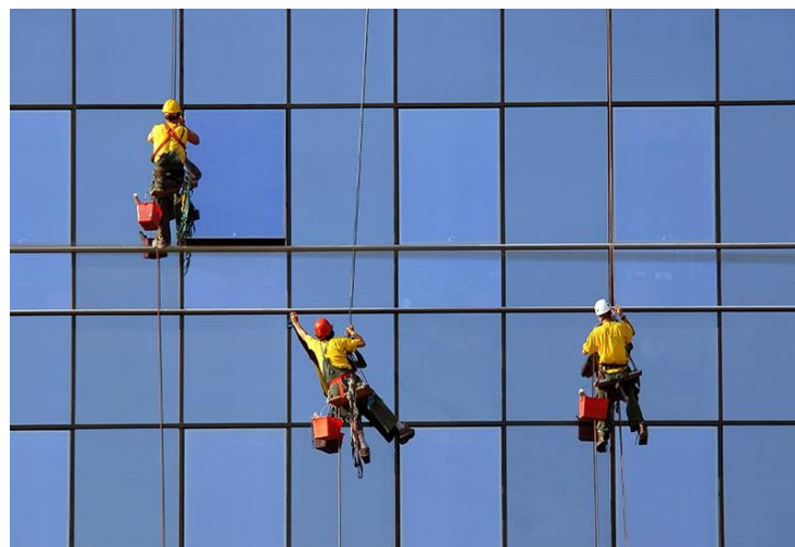
Figure 1: Workers cleaning windows by Abseiling Method
