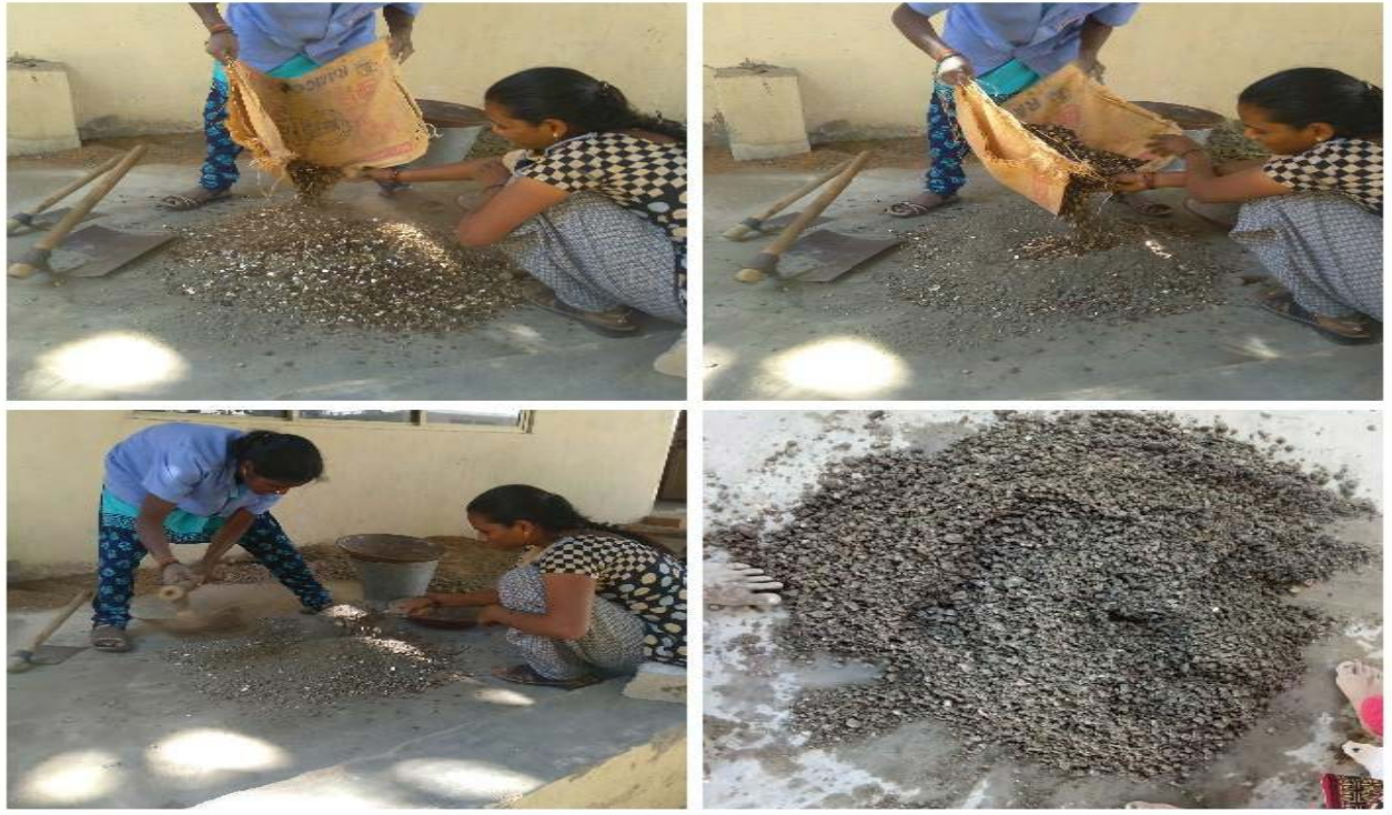
Fig 2:Mixing of Concrete
