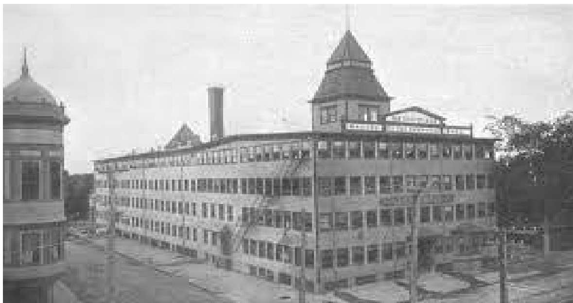
FIG 2.2 (a) GROOVER SHOE FACTORY BEFORE THE BOILEREXPLOSION ON 20 MARCH 1905
