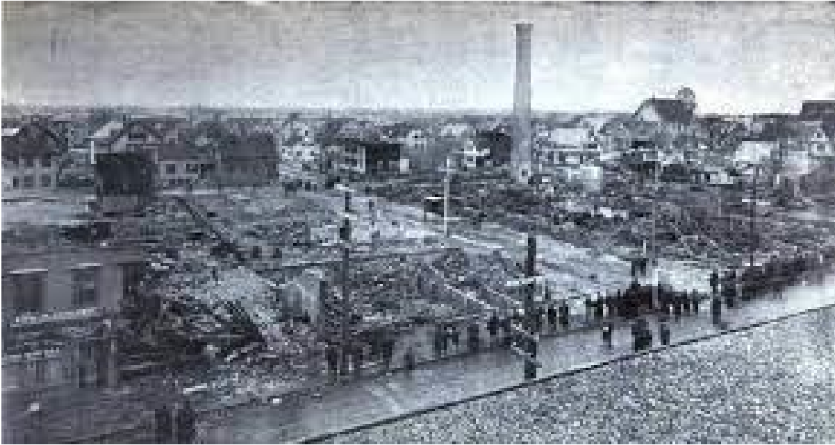
FIG 2.2 (b) GROOVER SHOE FACTORY AFTER THE BOILER EXPLOSION
