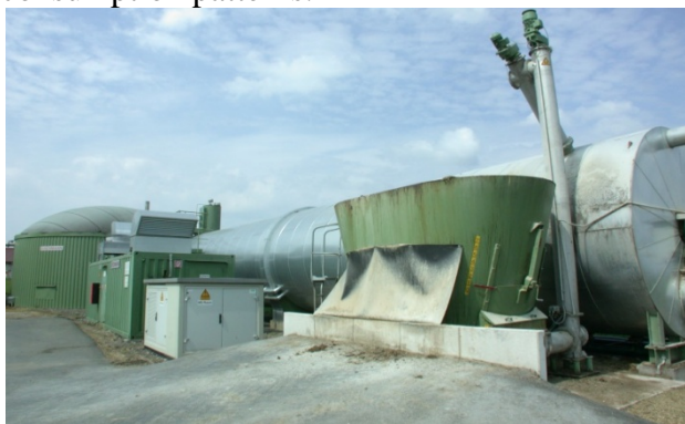
Fig.1 farmyard anaerobic digester converts waste plant material and manure from livestock into biogas fuel.
