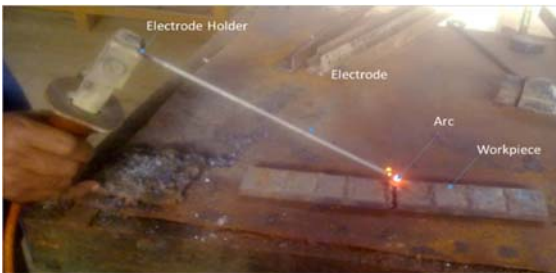
Fig.1.Electric Arc welding Process
